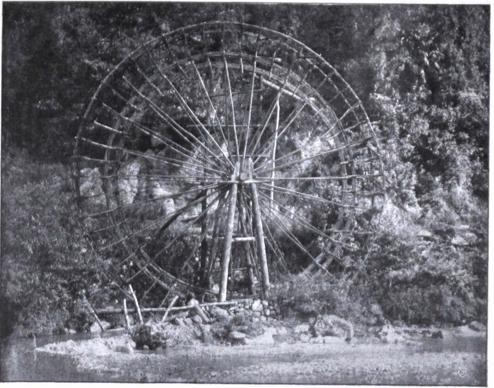
UNDERSHOT WATER-WHEEL (BAMBOO), USED FOR THE IRRIGATION OF RICEFIELDS, SZECHUAN.
